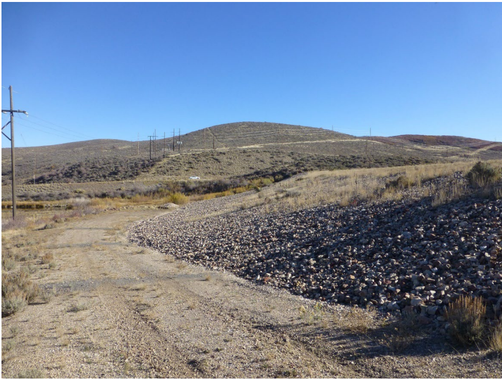
Toe of the main embankment
